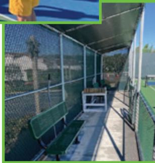
MARCH - Sports Clinic and Court Improvements
