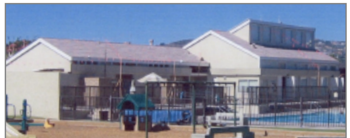
The MPR building that was
