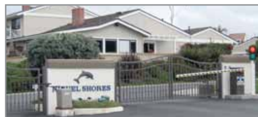
Manta Court Gate
