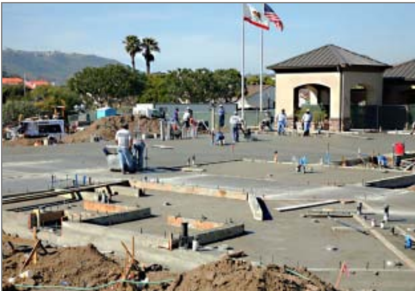
Cement was poured for the Clubhouse foundation on March 17. Photo by Gary Tinnes
