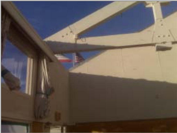
Our Multi-Purpose Room now in a state of demolition—we loved it for 35 years—see a tribute on page 8.
