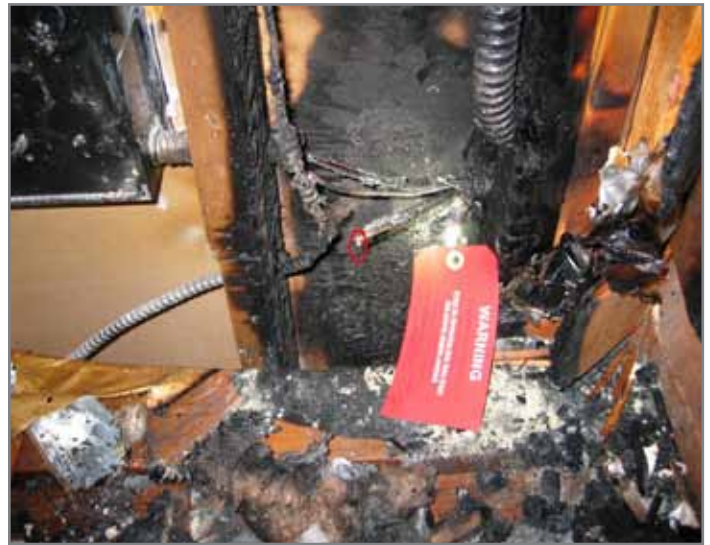
Fire damage in the men's sauna
