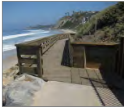
Crescent Walk along Strand Beach
